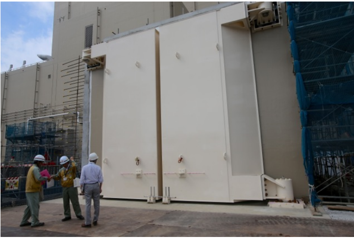
Photo 7. Doors now doubled on the reactor building
