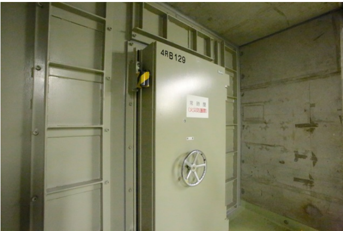
Photo 8. Watertight doors for critical areas
