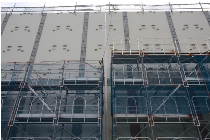
Photo 6. Massive 12-meter high seawall (front view)
