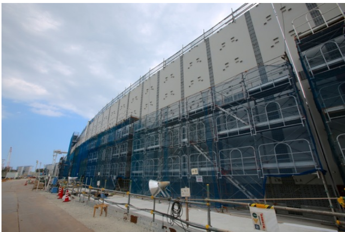
Photo 5. Massive 12-meter high seawall
