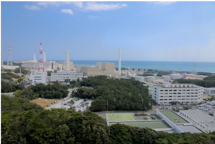
Photo 1. Full skyline view of Hamaoka Nuclear Power Station
