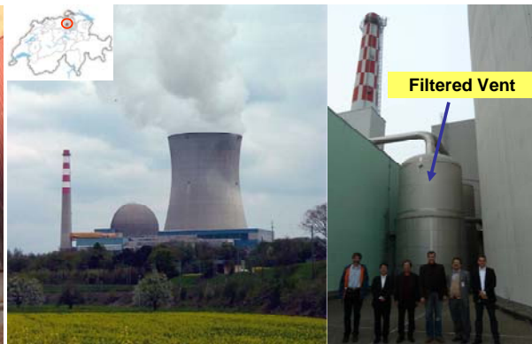
Fig. 17 FCVS in Leibstadt NPP, Switzerland
