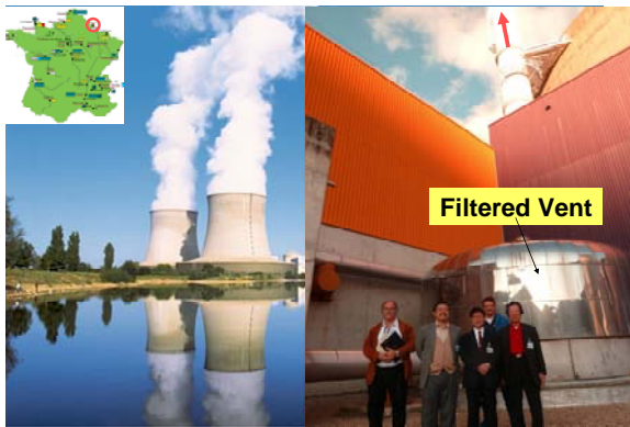
Fig. 16 Installed FCVS in Chooz NPP, France
